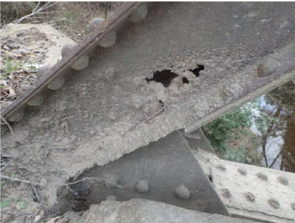
Photo 1: Truss End Post
