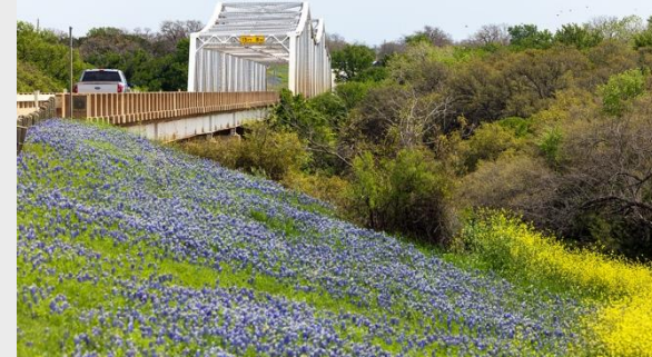
Truck approaching bridge
