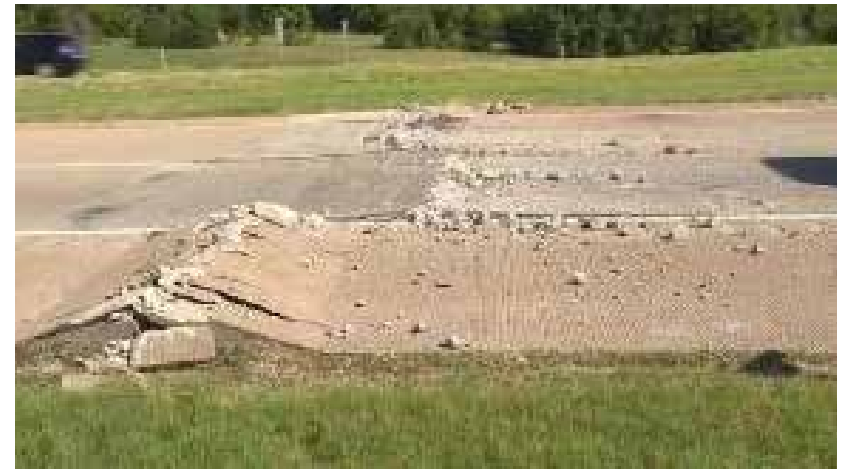
Road buckling from extreme heat on US Highway 75 southbound in Denison, Texas. July 2016.
