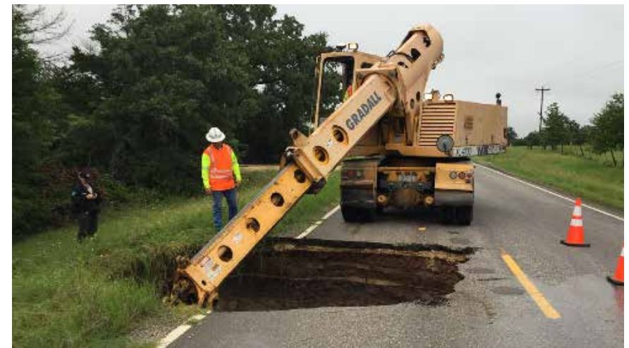
Sink hole in the road being fixed by a work crew.
