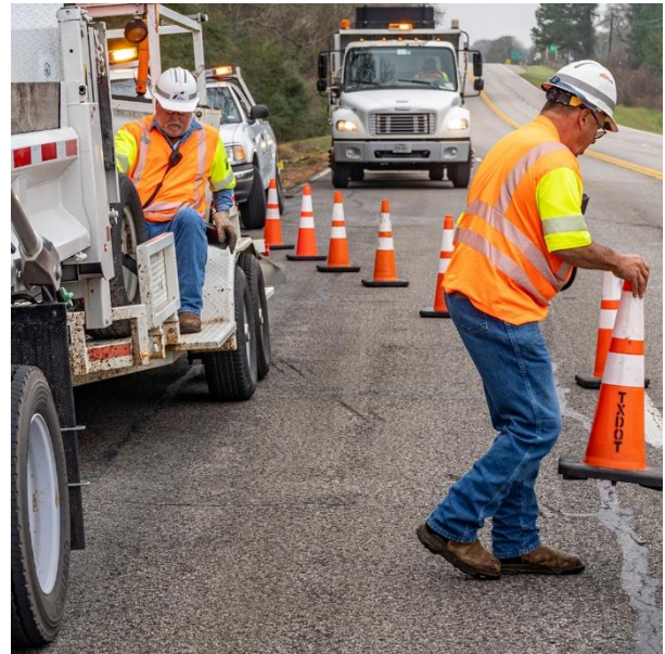
Figure 6: TxDOT Maintenance Crew
