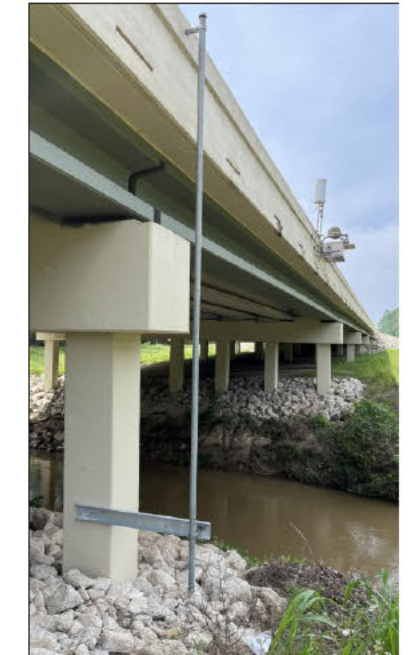
Typical Crest Stage Gage install
