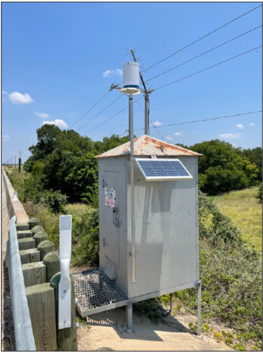
Typical installation of Step-In Type Gage Shelter on stand
