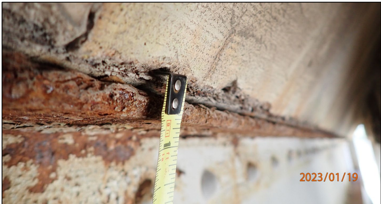
Figure 18 Floorbeam pack rust
