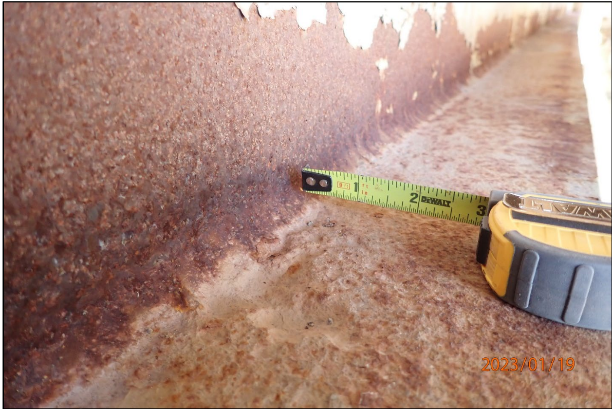
Figure 17 Floorbeam pitting
