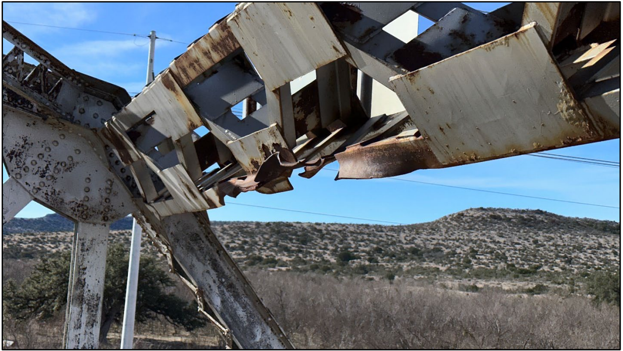
Figure 15 Portal bracing impact damage
