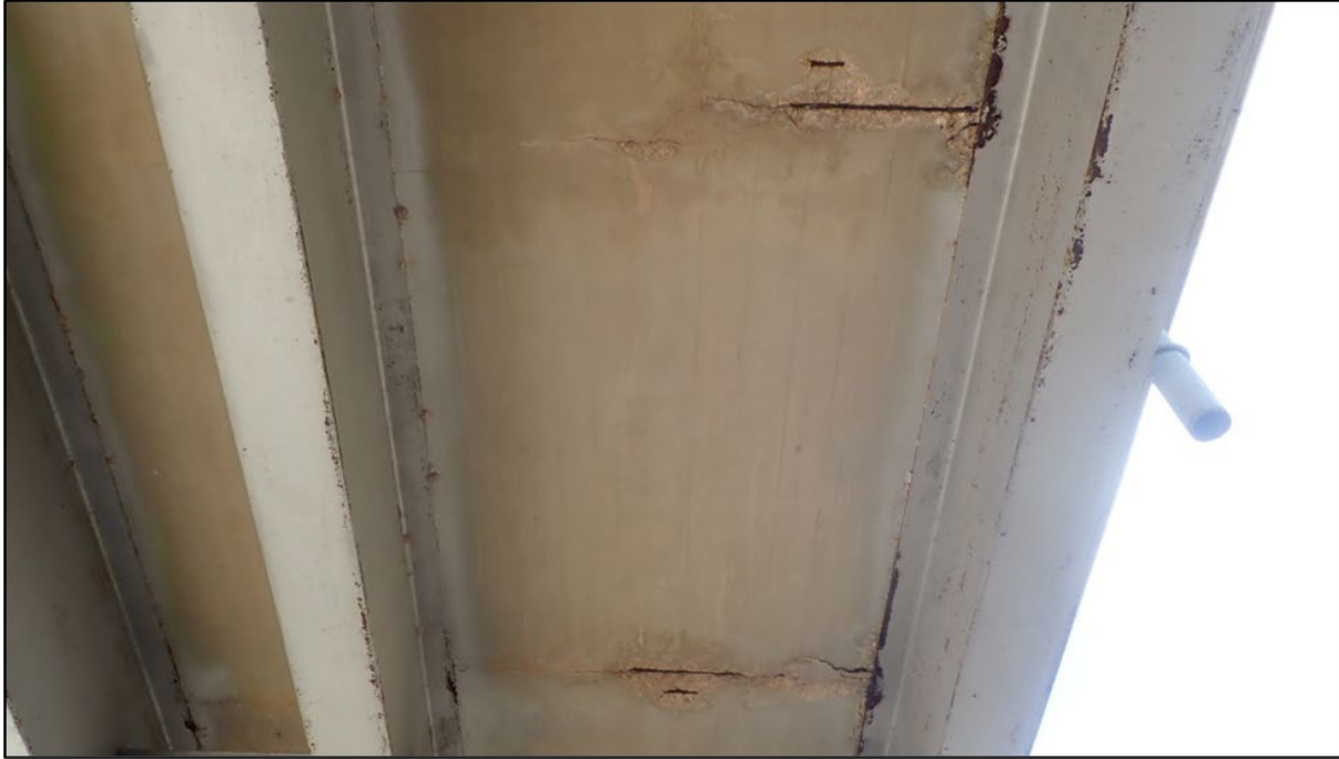
Figure 1 Spalls in deck soffit span
