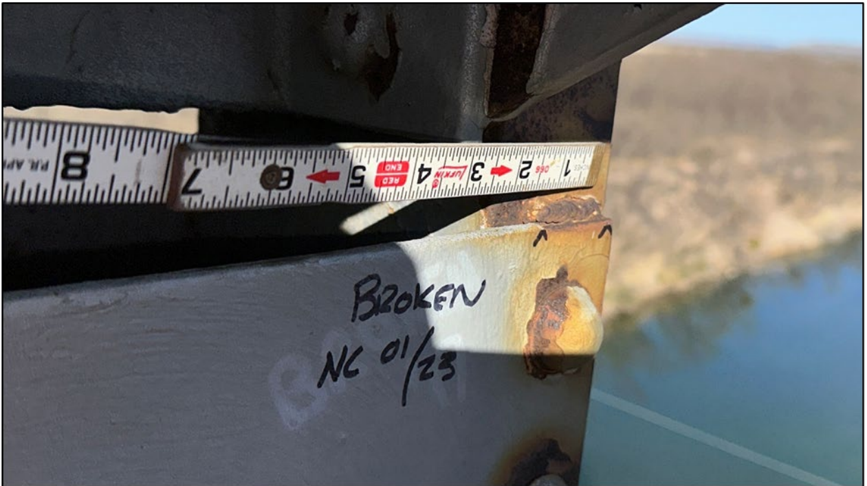
Figure 8 South truss batten plate
