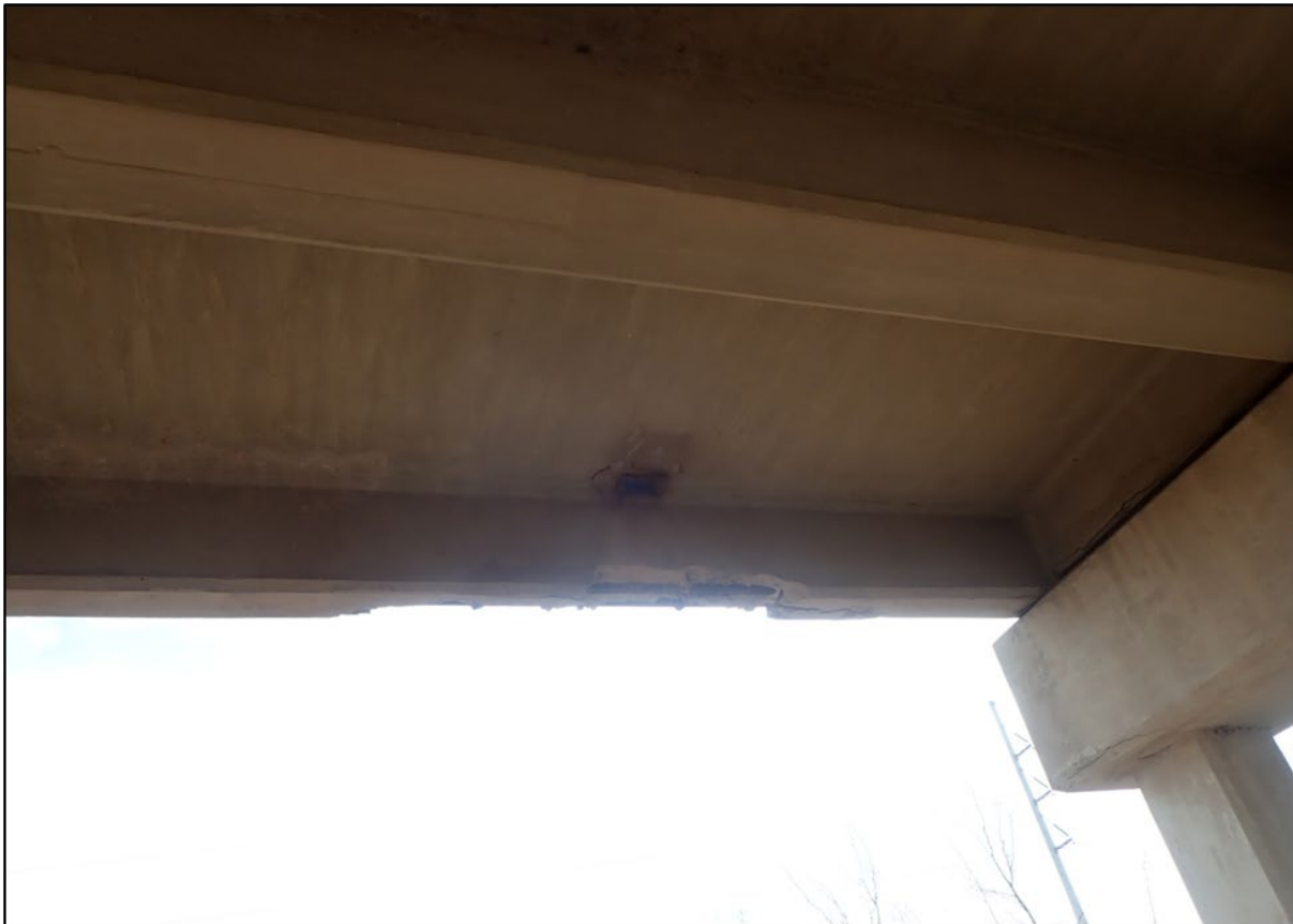
Figure 2 Spall in south beam span
