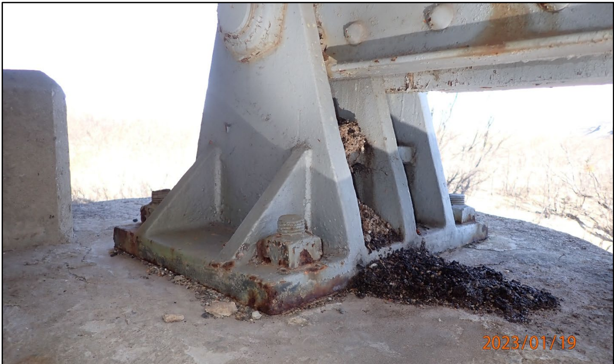
Figure 20 Truss bearing surface corrosion
