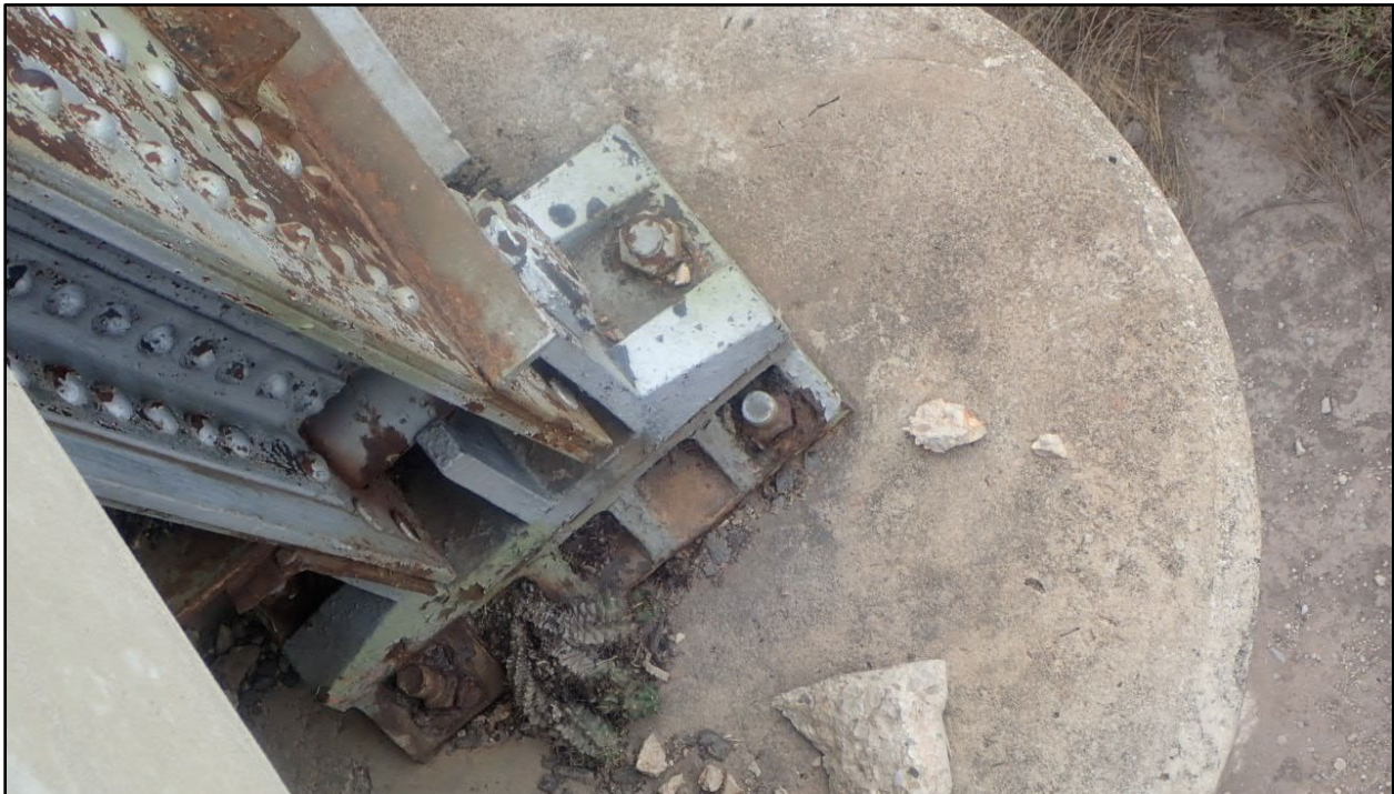
Figure 6 Rusted east bearing plate for truss bent
