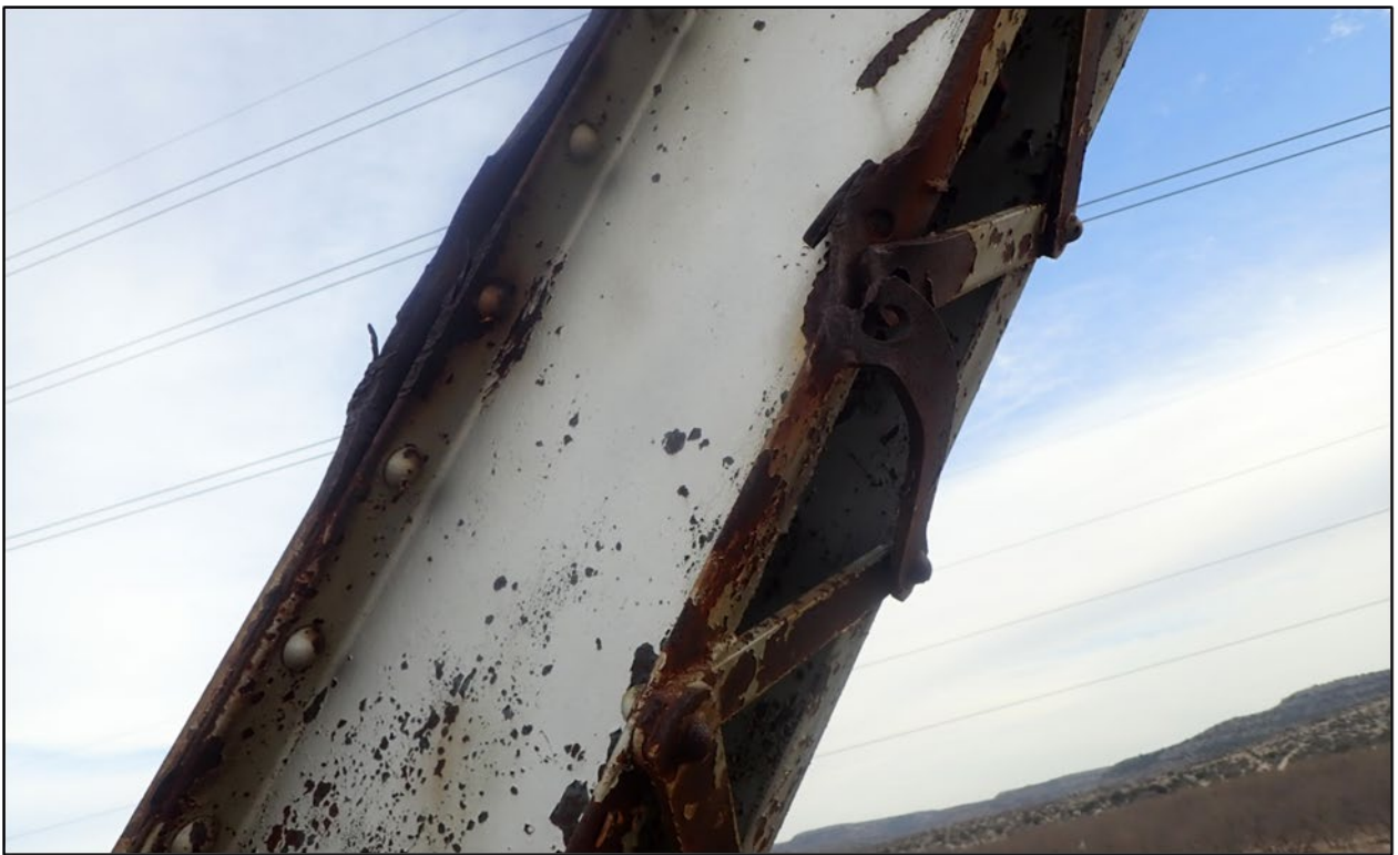
Figure 4 Impact damage south truss
