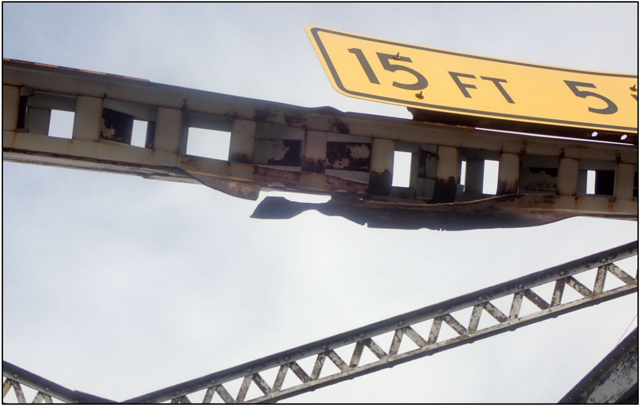
Figure 3 Impact damage on west horizontal
