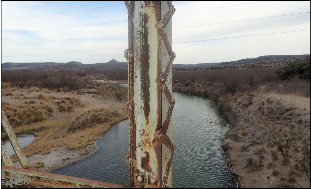
Figure 5 Impact damage south truss
