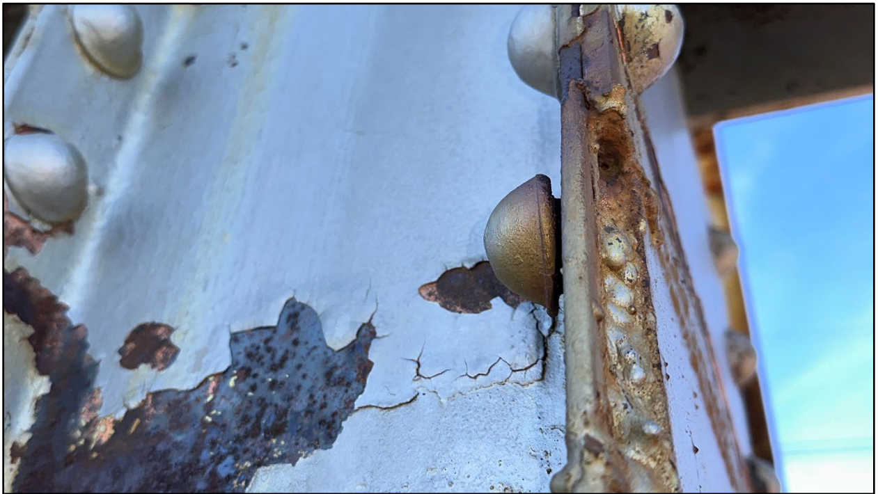
Figure 16 North truss unseated rivet
