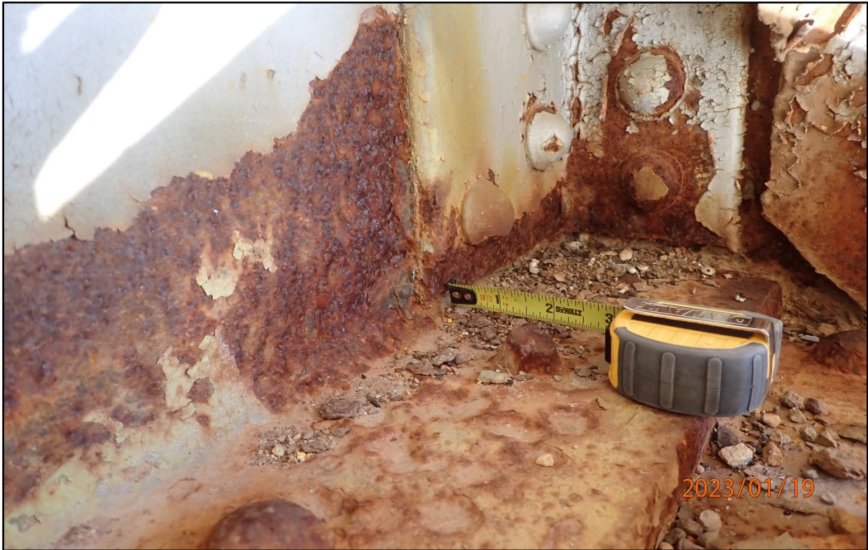
Figure 19 Floorbeam section loss
