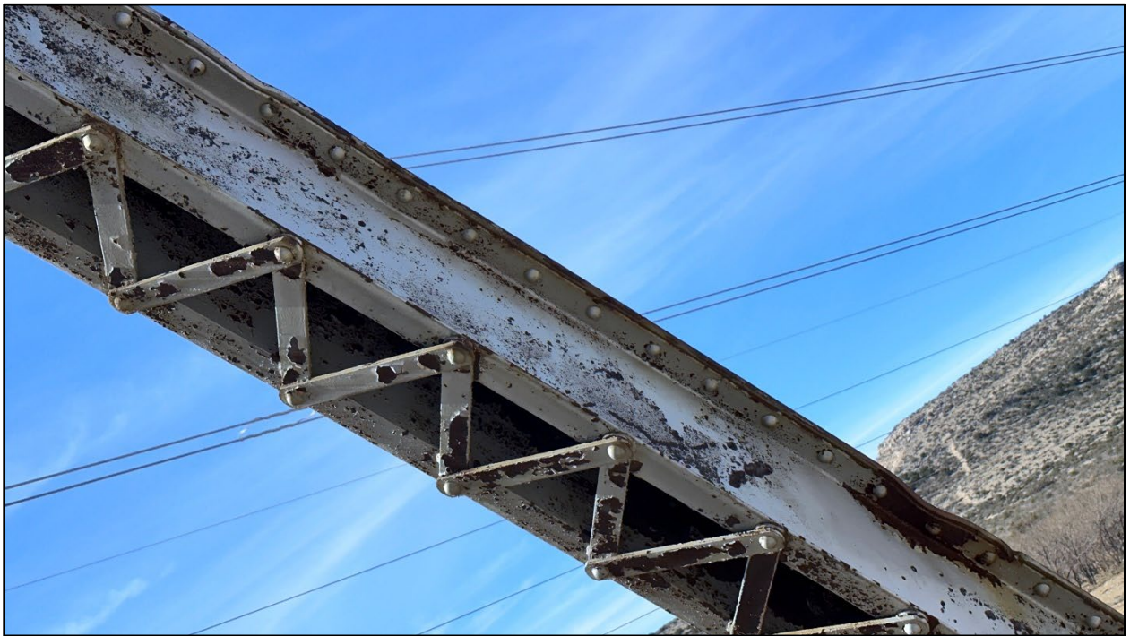
Figure 14 South truss impact damage
