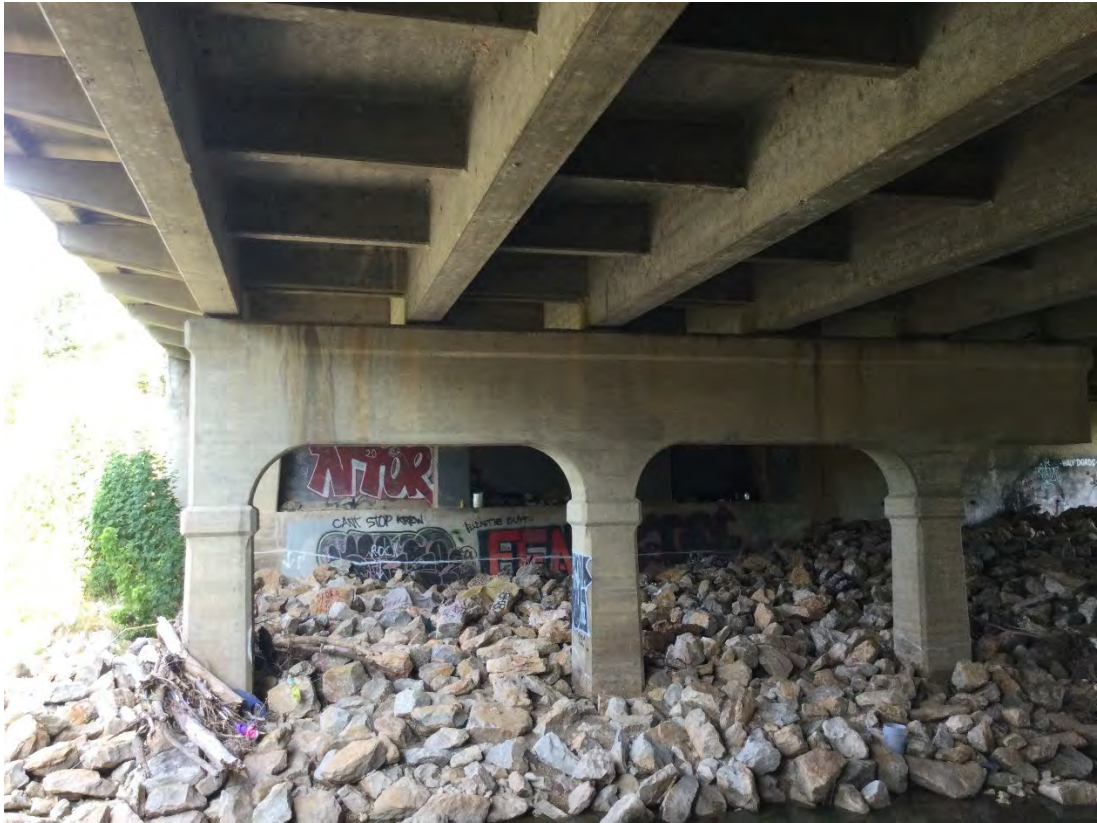
Figure 4. Underside of SH 180 bridge over Sycamore Creek, facing west. TxDOT
