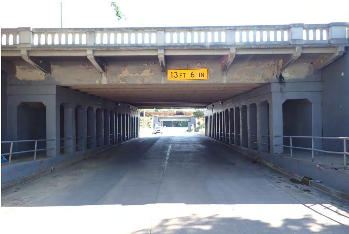
Figure 6. State Highway 180 bridge over Harwood Street, facing north. TxDOT
