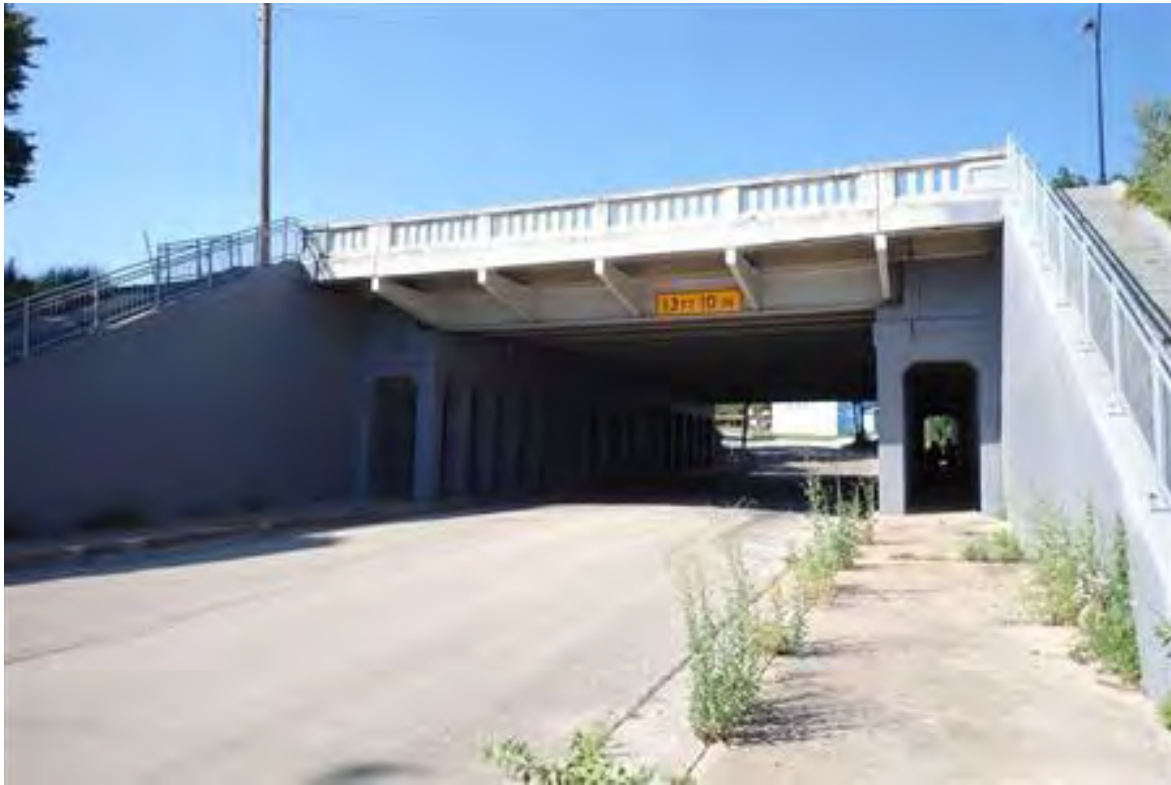
Figure 5. SH 180 bridge over Harwood Street, facing northwest. TxDOT
