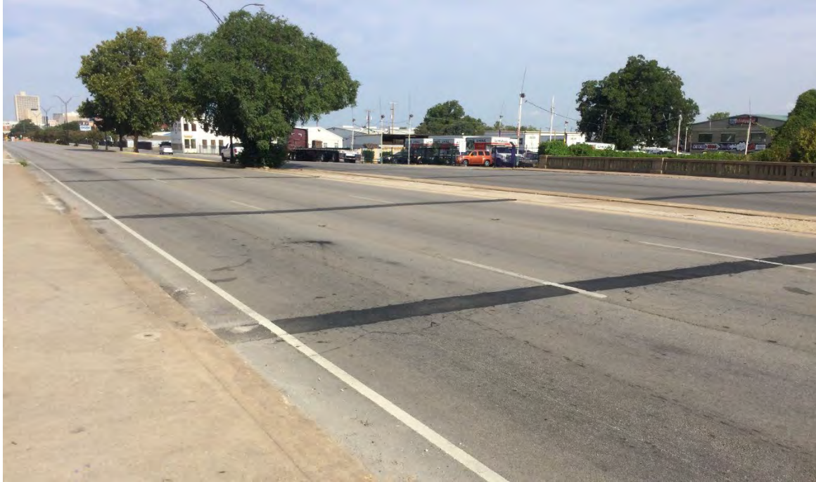
Figure 3. Road-level view of SH 180 over Sycamore Creek, looking west. TxDOT
