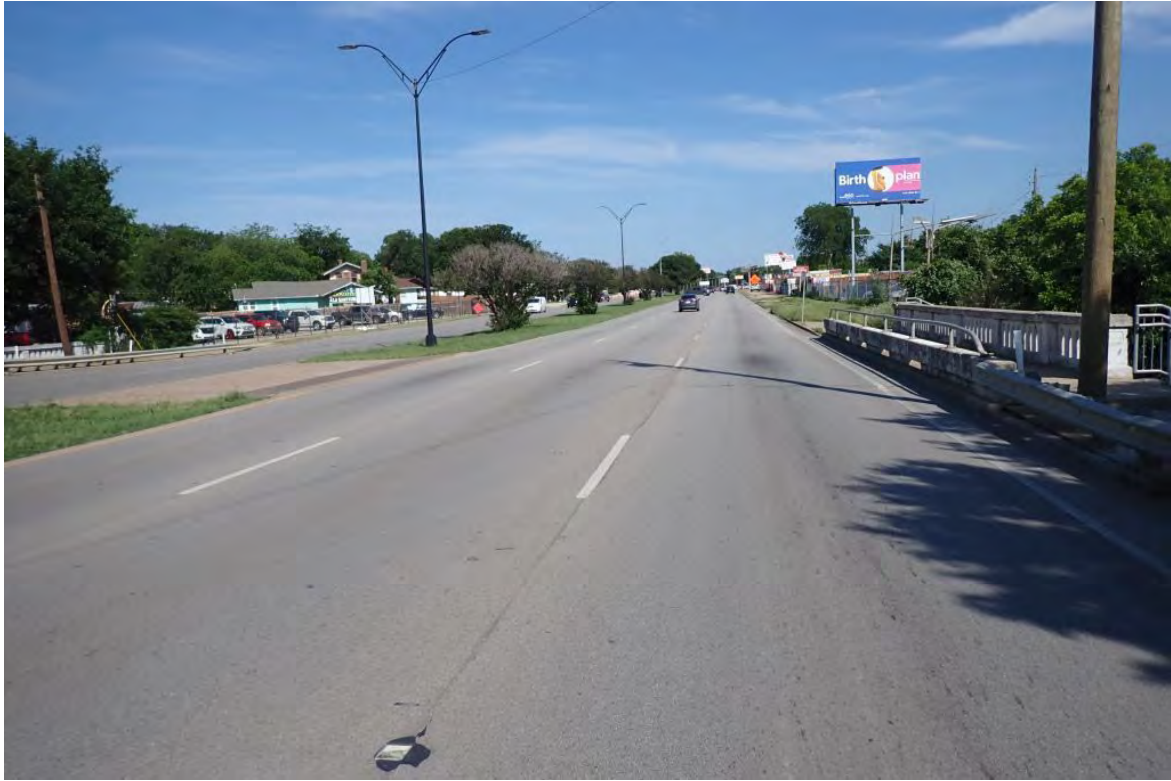
Figure 7. Street-level view of State Highway 180 over Harwood Street, facing southeast. TxDOT
