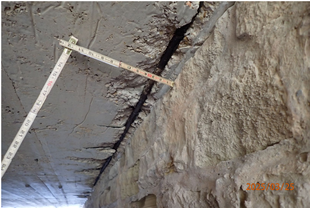
Figure 6. Abutment wall showing missing stones and vertical cracks.
