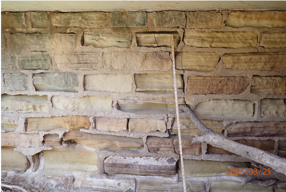
Figure 6. Abutment wall showing missing stones and vertical cracks.
