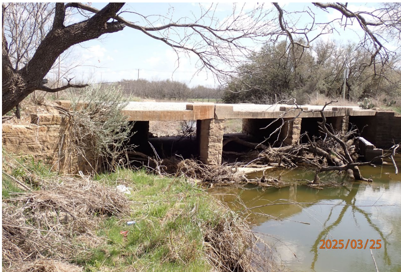
Figure 1. Side view of the bridge, facing east.
