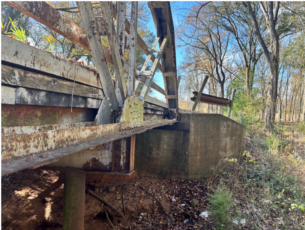
Figure 5. Side view of the CR 310 Bridge over Davidson Creek, looking to the south
