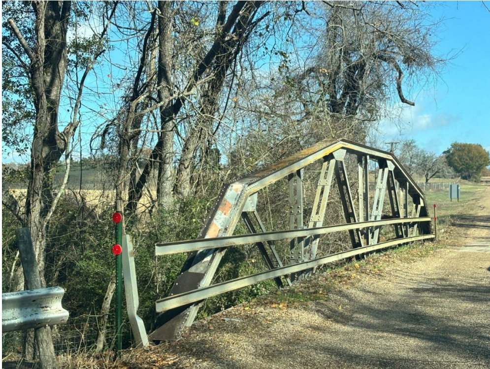
Figure 6. View of the bridge truss from the CR 310 roadway corridor, looking to the north.
