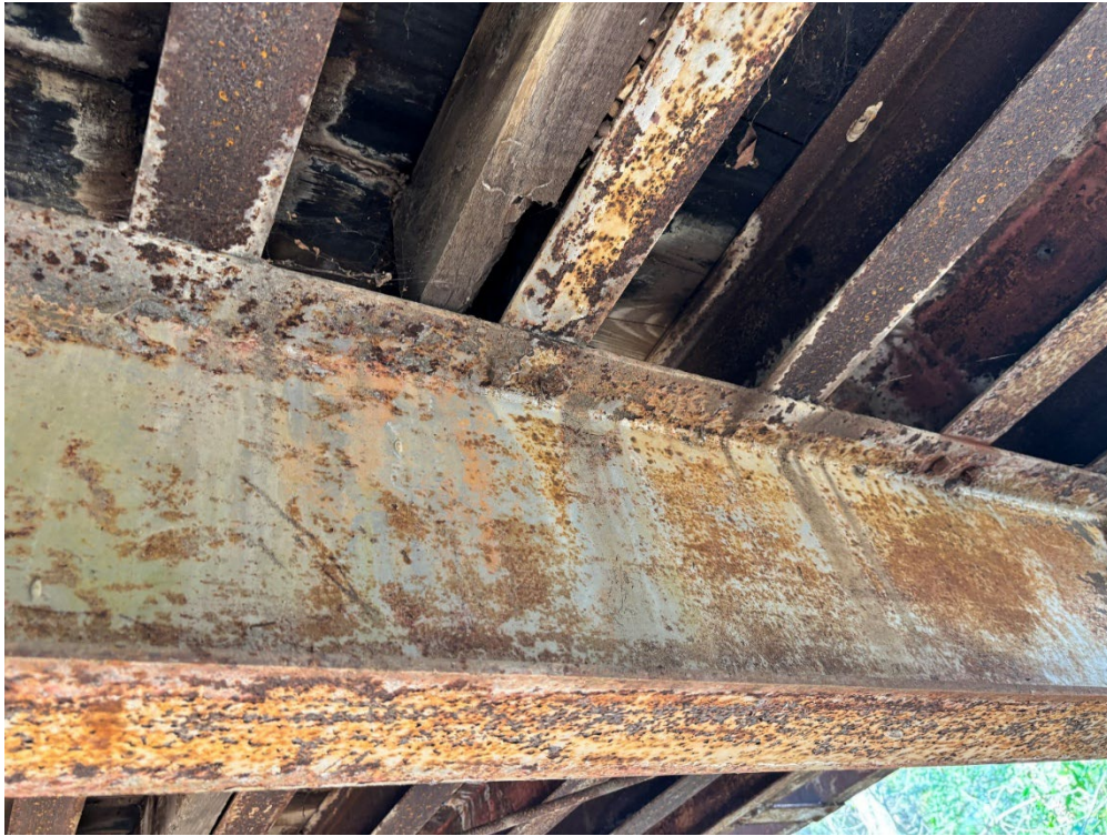
Figure 8. View of the bridge structure from the underside of the CR 310 bridge.
