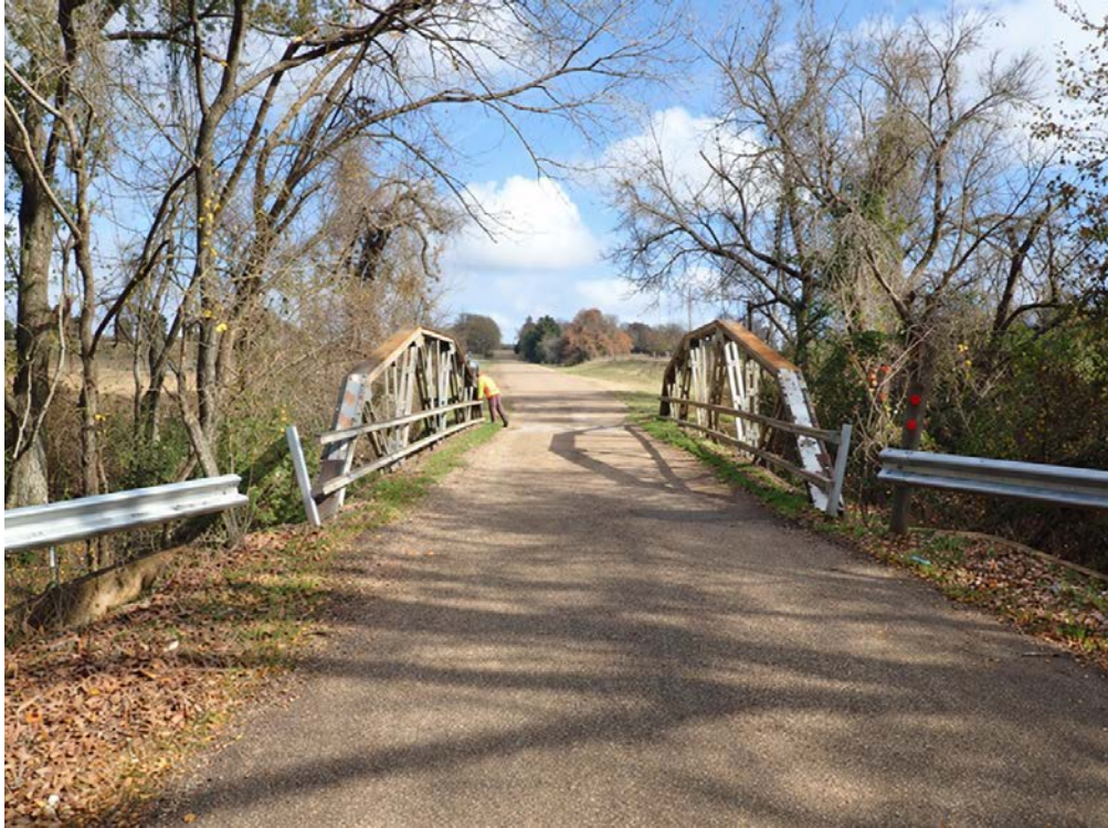
Figure 2. View of the CR 310 bridge over Davidson Creek from the roadway corridor looking to the northeast.
