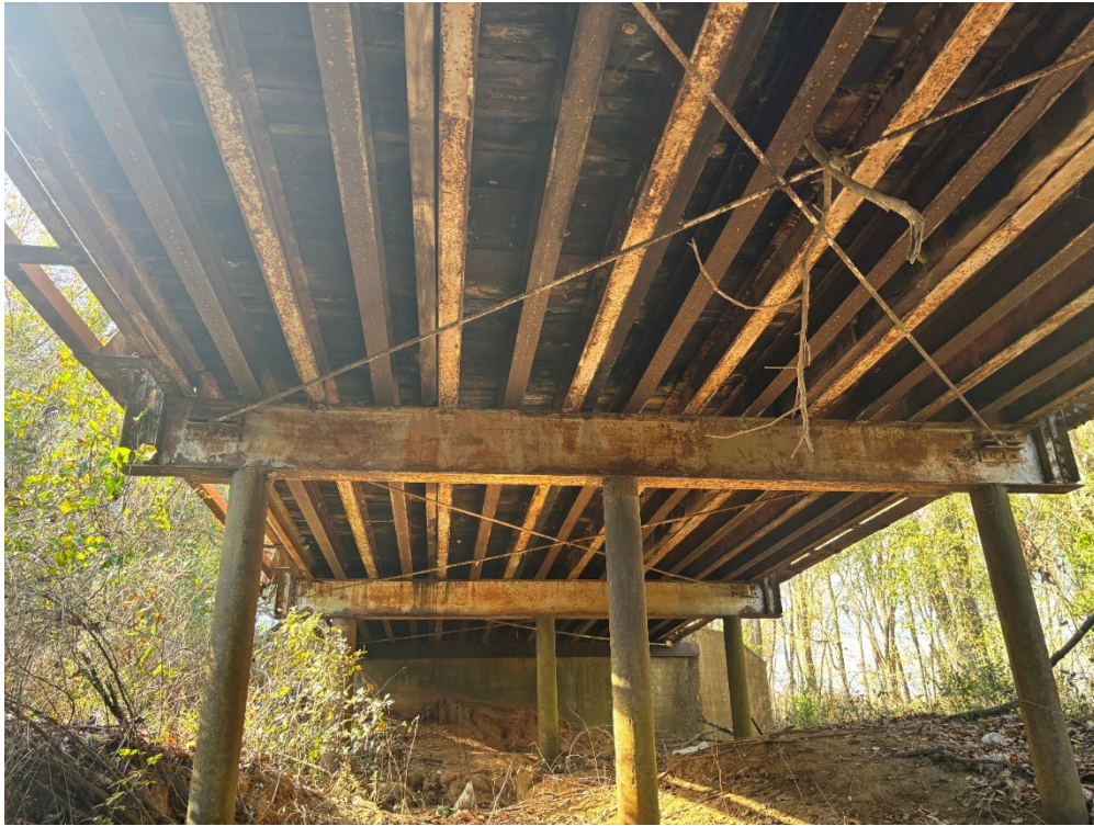
Figure 4. View of the bridge columns and abutment from the underside of the bridge, looking to the south.
