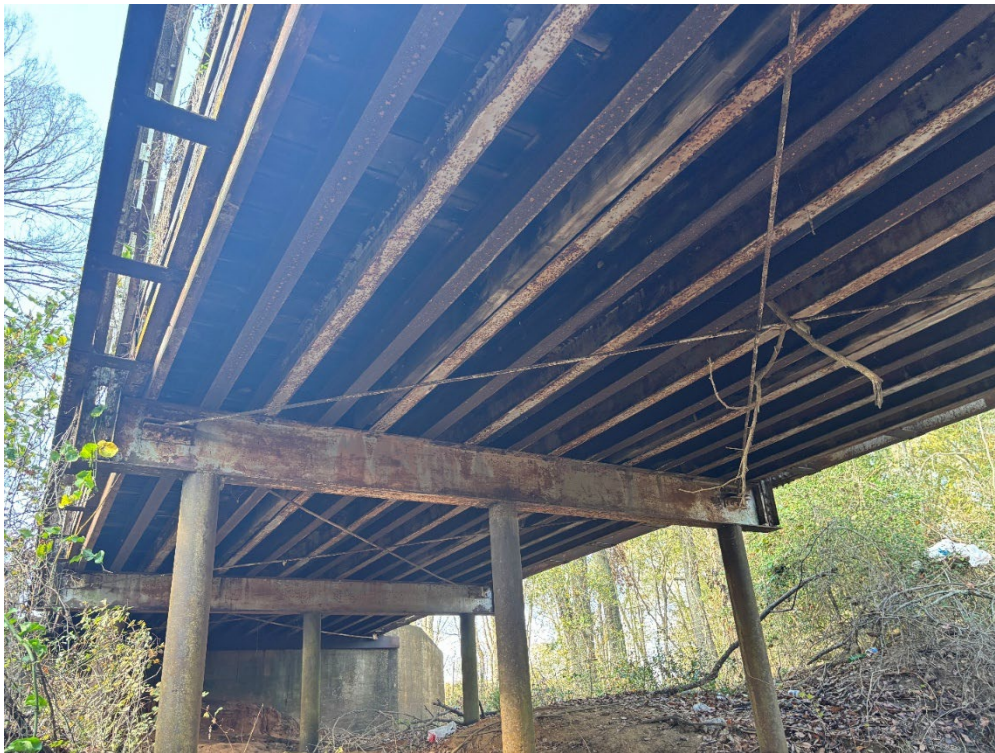
Figure 3. View of the underside of the bridge, looking to the southwest.
