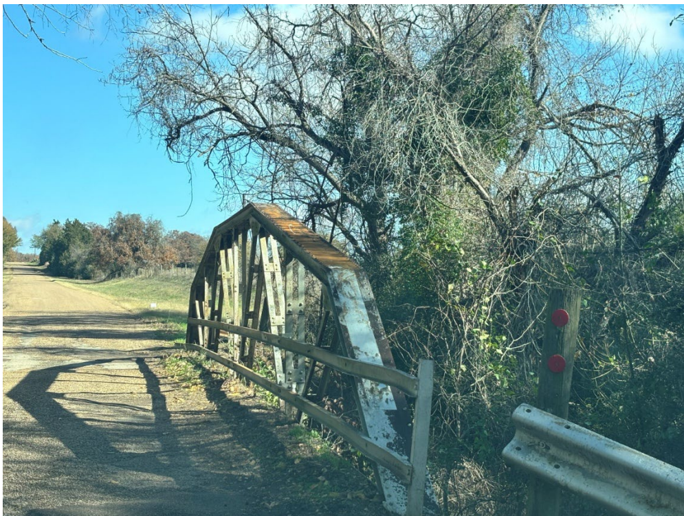
Figure 7. View of the bridge truss from the CR 310 roadway corridor, looking to the northeast.
