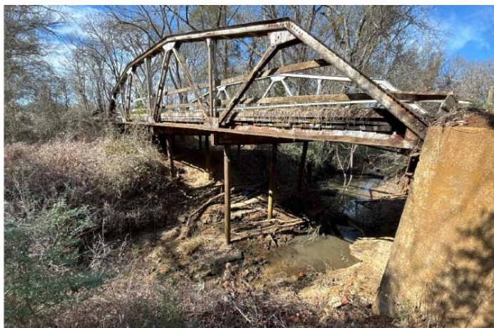
Figure 1. Side view of the CR 310 Bridge over Davidson Creek, looking to the southwest
