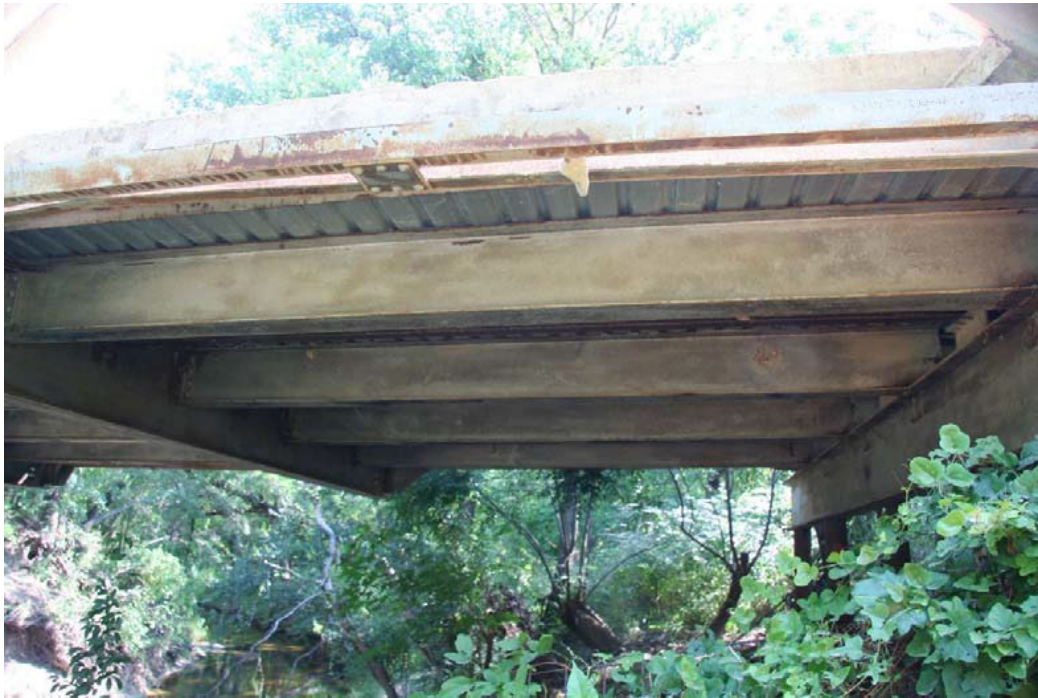
Figure 5. Underside of bridge, showing alterations to stringers and new bent
