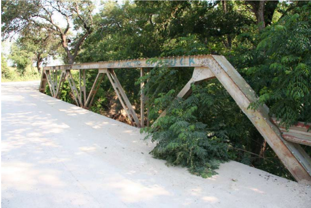
Figure 3. View of the east side of the bridge truss.
