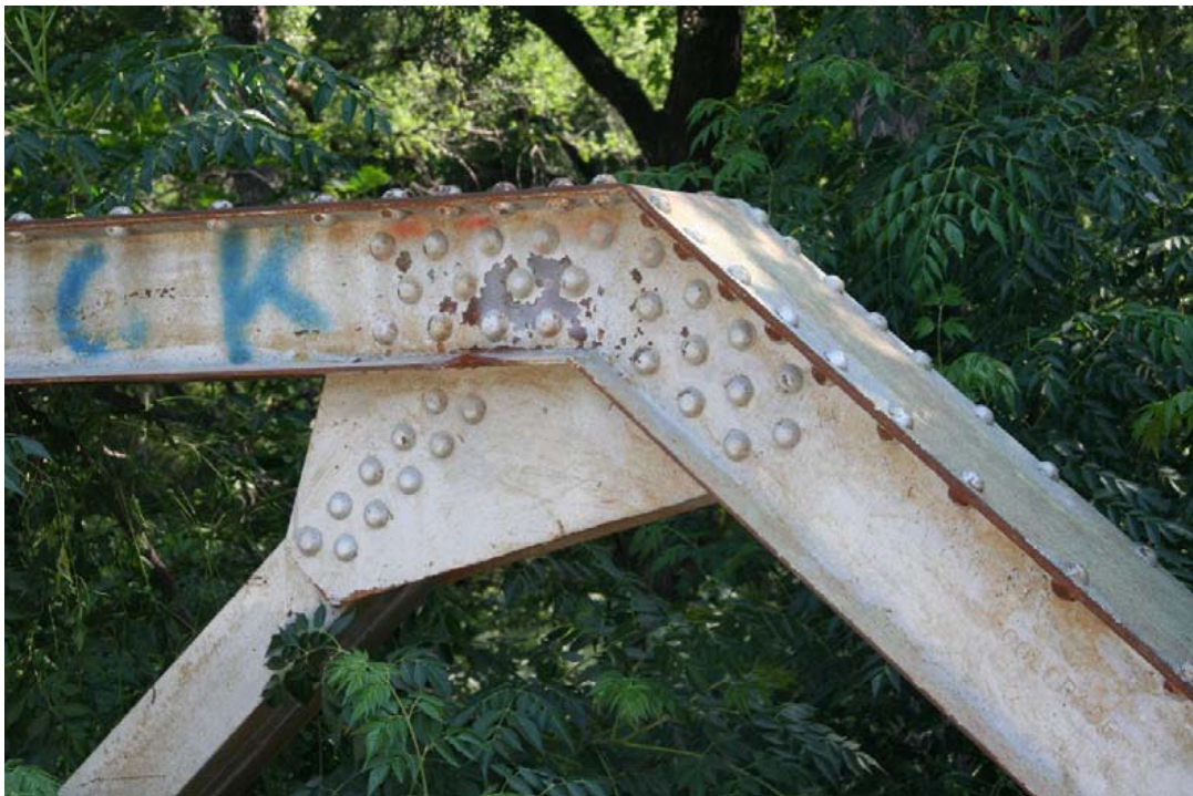
Figure 4. Detail of top chord connection
