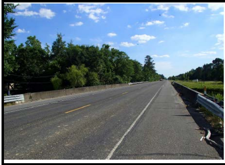
Appendix A – Photo 1: Roadway View Over Bridge (facing SW)
