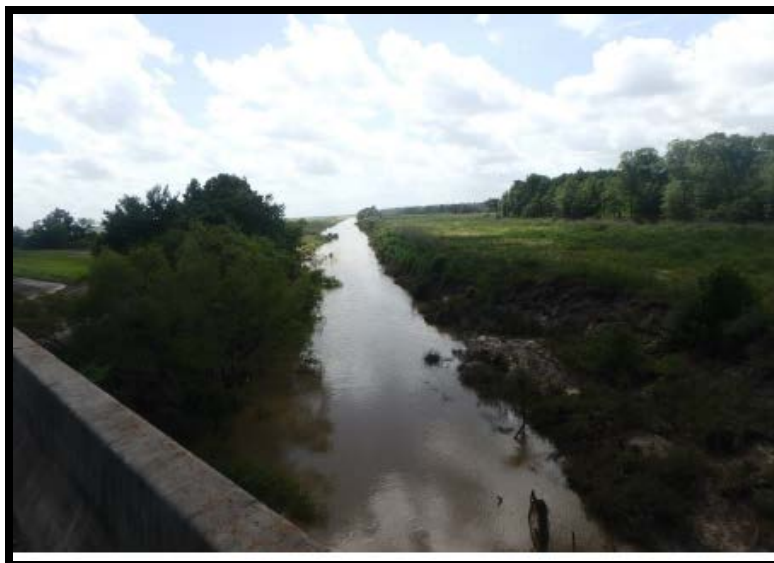
Appendix B – Photo 3: Upstream view of N Fork Taylor Bayou from bridge at IH-10
