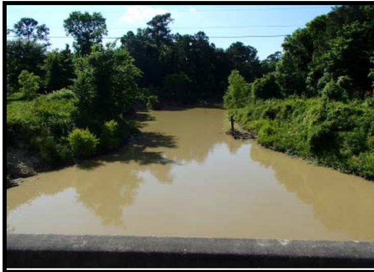
Appendix A – Photo 2: Upstream View From Bridge
