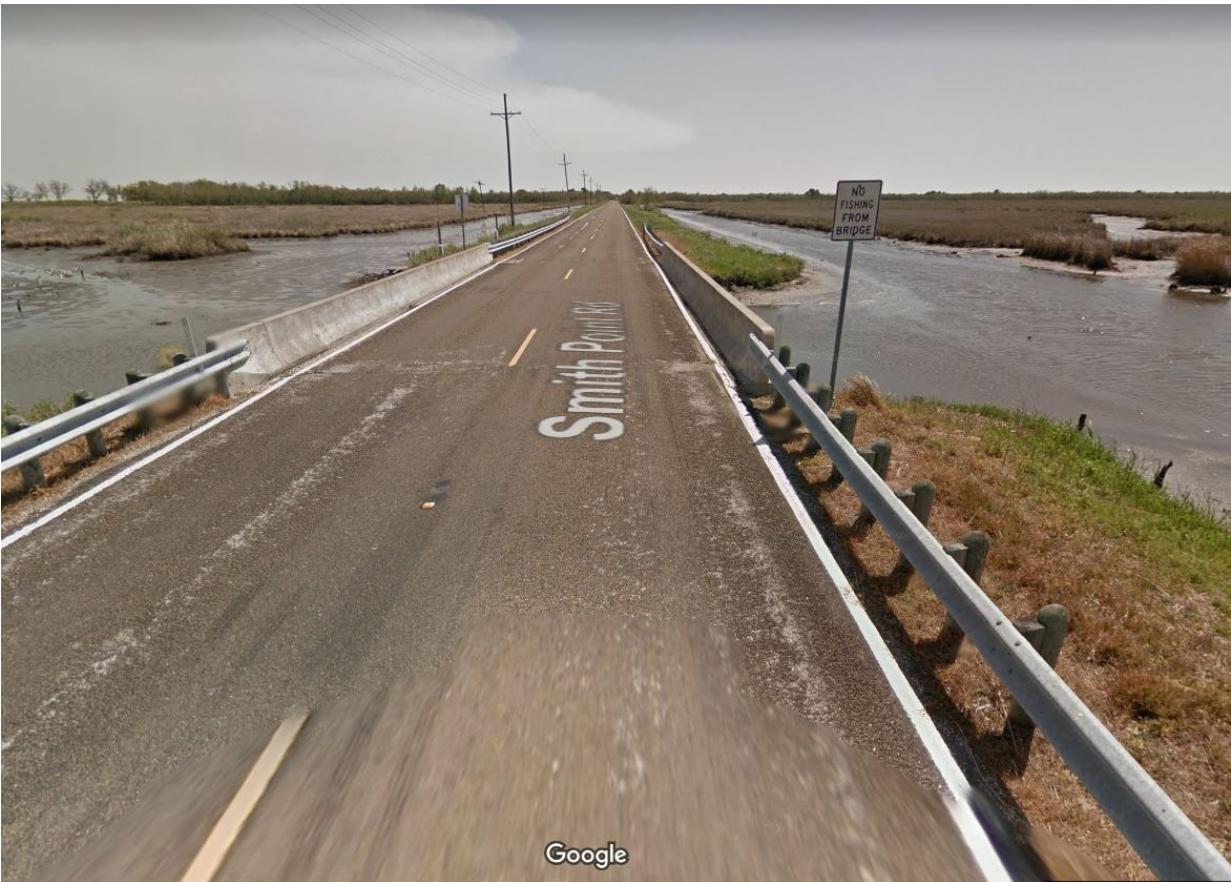
Photo 4. Lone Oak Bayou at the FM 562 bridge, facing south.
