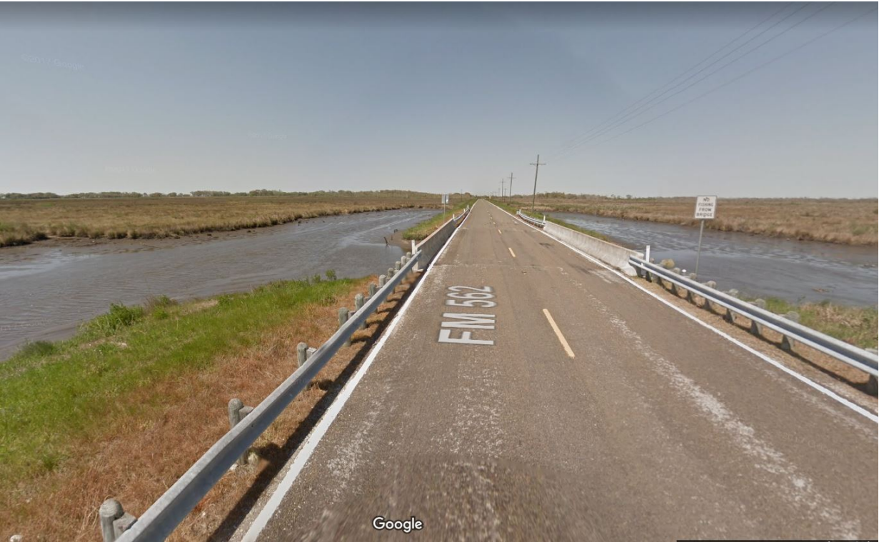
Photo 3. Lone Oak Bayou at the FM 562 bridge, facing north.
