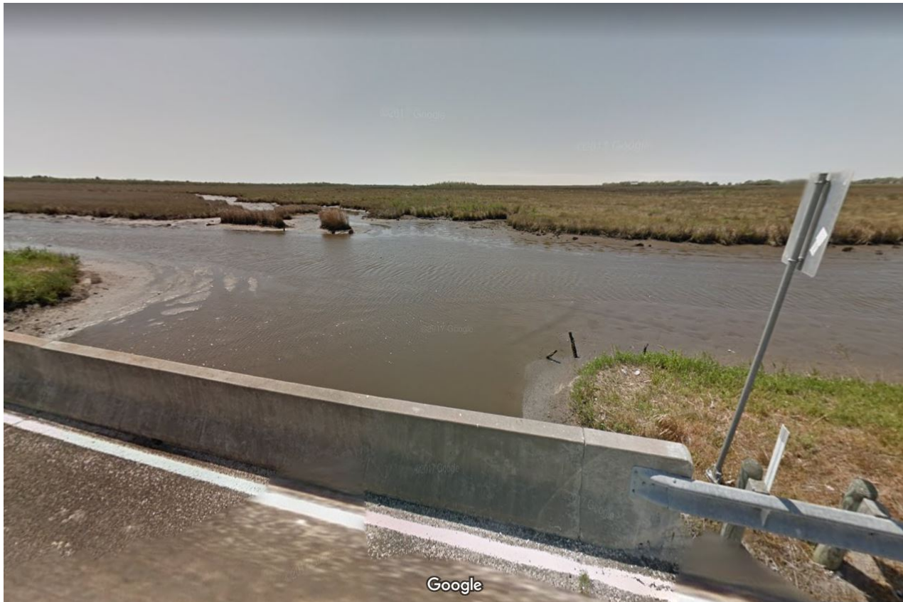
Photo 2. Lone Oak Bayou at the FM 562 bridge, facing west.
