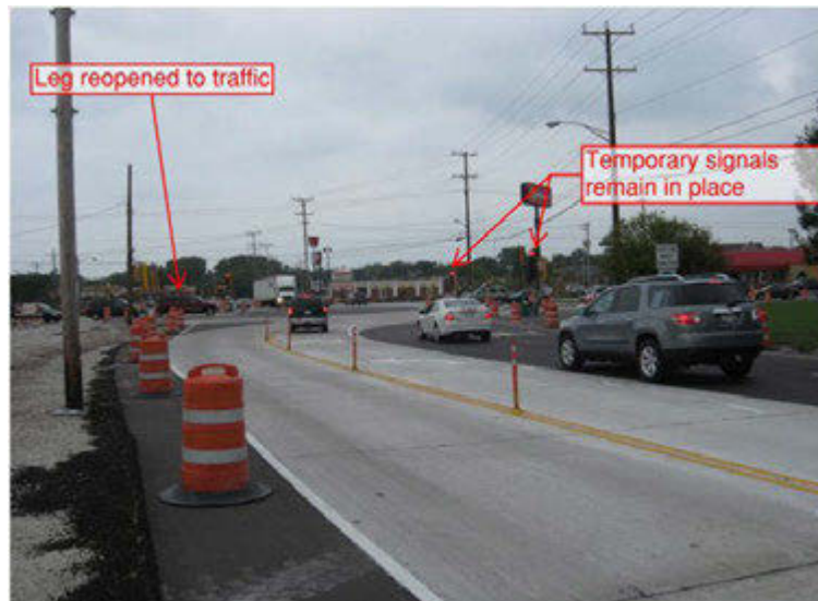
» EXAMPLE 5 – TEMP. TRAFFIC SIGNAL TIMINGS FOR PIECE-WORK WITH PAVE-THRU CONCEPT
