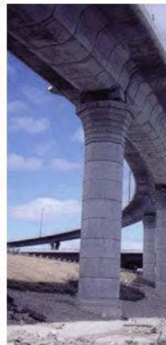
(b) Precast segmental column
