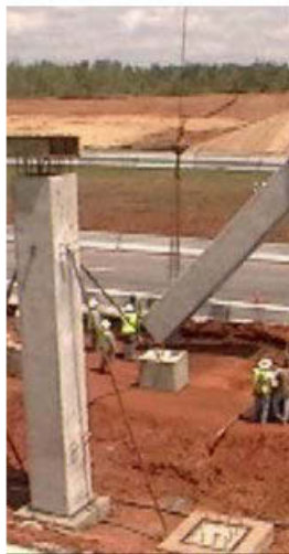
(a) Full-height precast column
