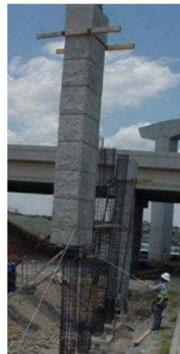
(c) Precast column shell
