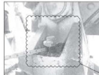
SPAN 8 NEAR TRUSS #1 AT LO (BENT 8)
