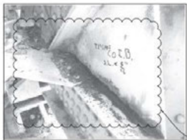
SPAN 10 TRUSS #1 AT L0 ①
