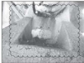
SPAN 7 NEAR TRUSS #2 AT LO (BENT 8)
