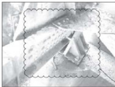
SPAN 10 TRUSS #1 AT L8 ①
