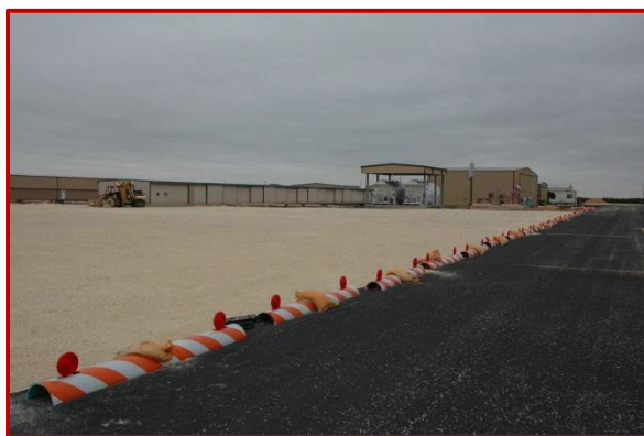
Figure 1. Construction at T.P. McCampbell Airport in Ingleside.
