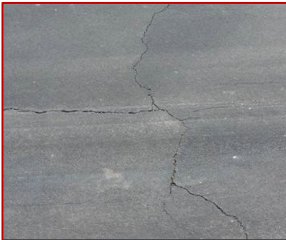
Figure 3. Pavement exhibiting cracking.
