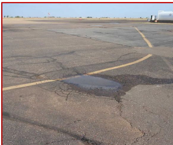
Figure 4. Poor drainage.
