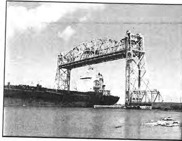
Tule Lake Lift Bridge
