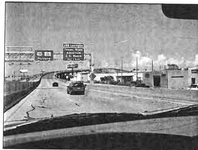
South end approach to Harbor Bridge.
