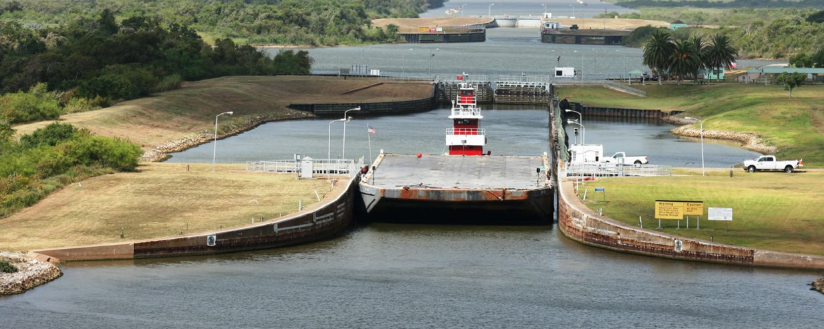
A 72-foot-wide barge navigates through the USACE Galveston District's 75-foot-wide Colorado River Locks in Matagorda, Texas. (Photo credit: USACE)
