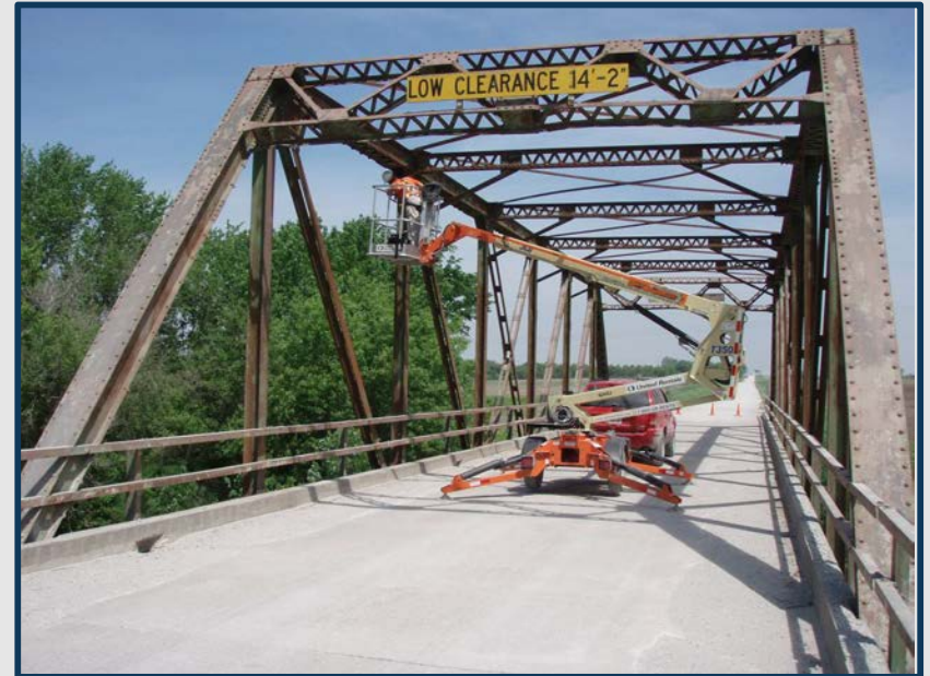
NSTM condition assessment with a Manlift
