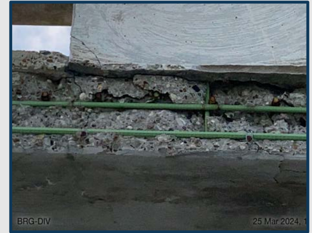
Concrete Spalling
