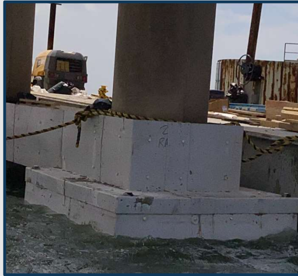
Cathodic Protection Assessment for Coastal Bridge
