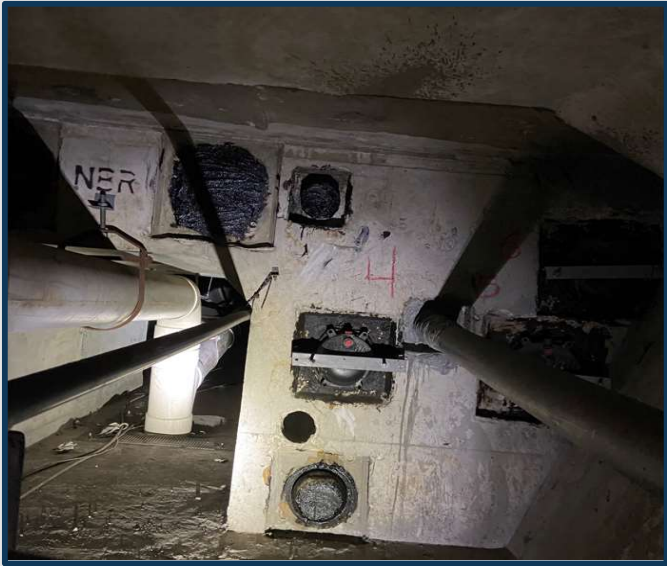
Condition Assessment of a Segmental Bridge
