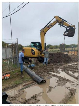
Patterson on site welding the 18" split casing
