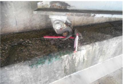
Figure 6-13. Example of rocker bearing requiring replacement
