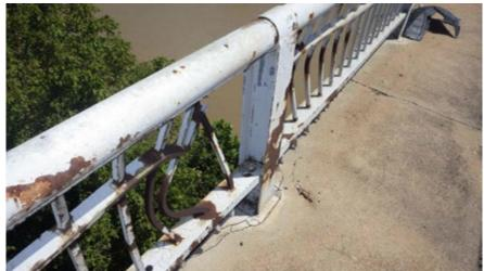
Figure 9-1: Damaged Type PR-1 (MOD) railing.
