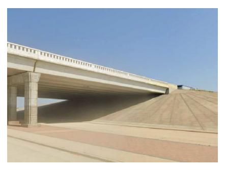
Figure 13-1: Concrete Riprap under Bridge Abutment
