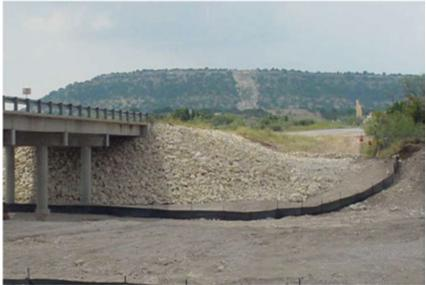
Figure 13-20: Stone Protection Riprap – Erosion at Toe
