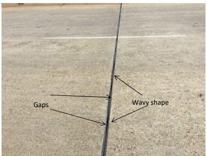
Figure 3-9: Deformed joint armors probably due to anchorage corrosion.
