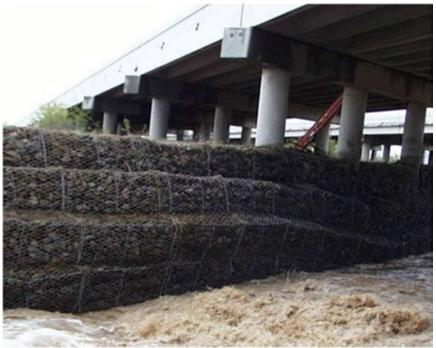
Figure 13-23: Gabions – Undermining and Settlement
