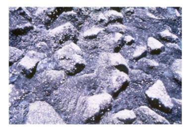
Figure 13-2: Grouted Stone Protection – Rough Surface
