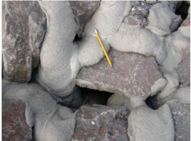
Figure 13-10: Partially Grouted Riprap – Close-up View
