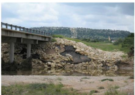
Figure 13-21: Stone Protection Riprap Compromised
