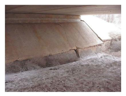
Figure 13-4: Concrete Riprap – Undermining at Toe. Note that the current CRR standard required a deeper toe than shown here.
