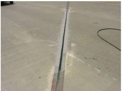
Figure 3-12: Example of partial elimination of armor joint.
