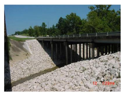
Figure 13-8: Stone Protection Riprap at Bridge Abutment and Pier
