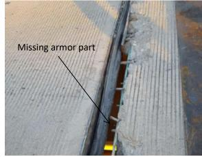
Figure 3-10: Example of a failed joint.
