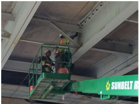
Figure 6-11. Installation of Post-Installed Shear Connectors.
