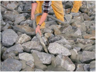
Figure 13-9: Partially Grouted Riprap
