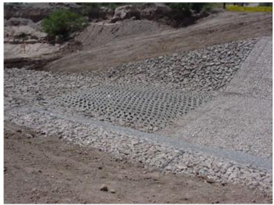
Figure 13-19: (Left to Right) Stone Protection Riprap, Articulated Concrete Armor Unit and Gabion Mattresses
