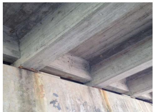
Figure 4-6: Lead sheet Slip.
