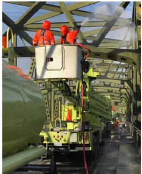
Figure 2-5: Bridge Deck Washing (Source: FHWA Bridge Preservation Guide)
