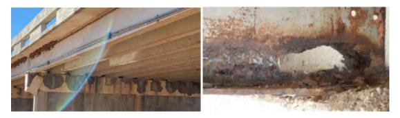
Figure 3-1: (a) Cap face spalling due to restricted movement; (b) Severe web corrosion due to debris build up on cap.
