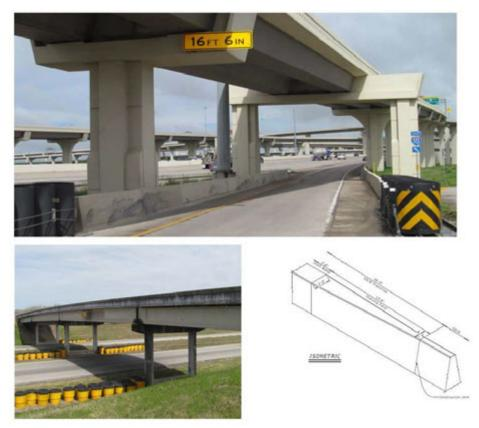
Figure 7-4. Various End Treatment Options. Top: Crash Cushion Attenuators; Left: Sand Barrel system; Right: Transition to concrete barrier
