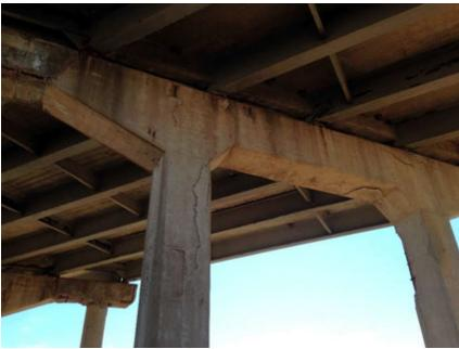
Figure 7-1. Example of concrete substructure deterioration.
