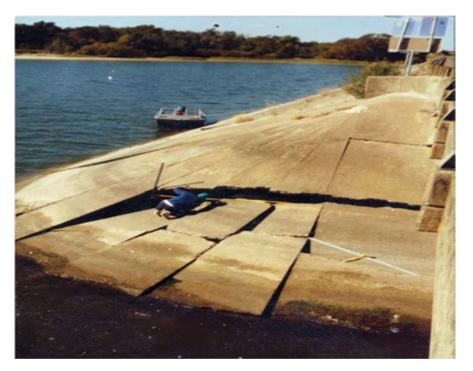
Figure 13-6: Concrete Riprap - Settlement Cracks
