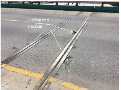
Figure 3-8: Loose joint due to concrete deterioration in anchorage areas.
