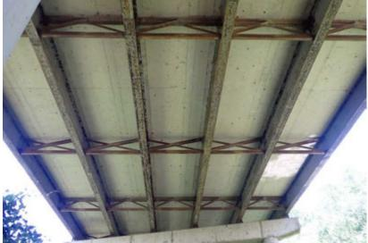
Figure 6-2: Paint failure of steel beams.
