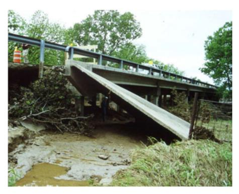
Figure 13-7: Concrete Riprap - Loss of Supporting Soil
