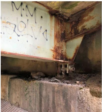
Figure 6-3: Corroded steel bearings under expansion joints.
