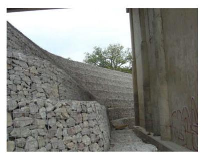
Figure 13-13: Gabions - Channel Bank Protection
