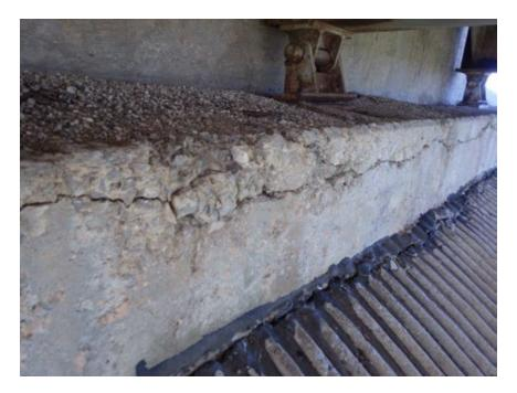
Figure 6-12. Example of rocker shoes requiring resetting, but not replacement.
