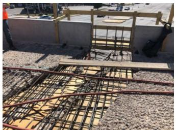
Figure 2-4: Full depth deck removal and reconstruction at bridge joint due to advanced deterioration of deck at joint.
