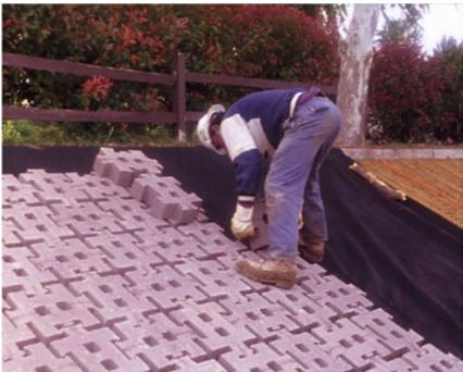
Figure 13-11: Interlocking Articulated Concrete Blocks
