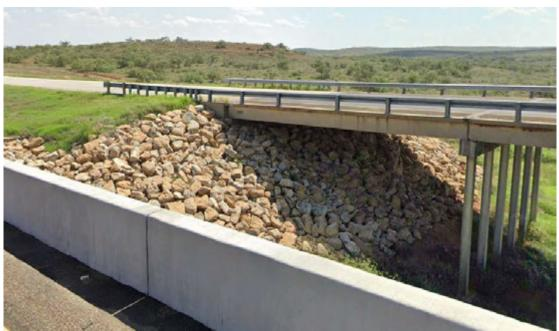
Figure 13-24: SRR used to replace a failed CRR.
