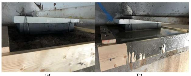
Figure 6-14. (a) Suspended sole bearing pad from sole plate with surface preparation and (b) Casting of bearing seat to obtain bearing at proper elevation.
