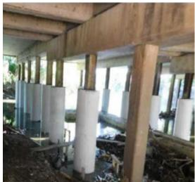
Figure 8-2. Steel piling with concrete encasements installed to address severe steel section loss.
