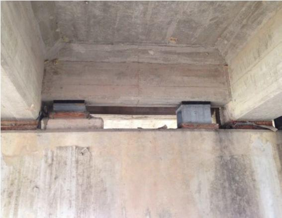
Figure 4-4: Pedestals used to retrofit T-beam end cracking.
