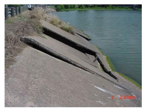
Figure 13-5: Concrete Riprap - Undermining and Settlement
