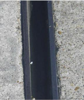
An example of a poured silicone seal is shown in Figure 3-6.
