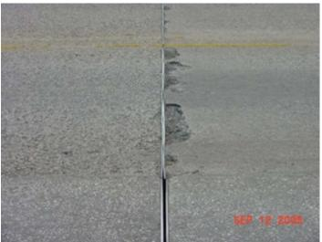
Figure 3-11: Example of closed-up armor joint.
