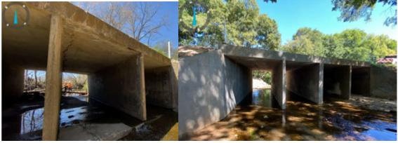
(a) (b) Figure 10-1: (a) Culvert Failure due to Undermining; (b) Failed boxed replaced in-kind
