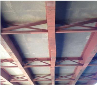
Figure 6-1: Over-height vehicle impact damage to steel beams.
