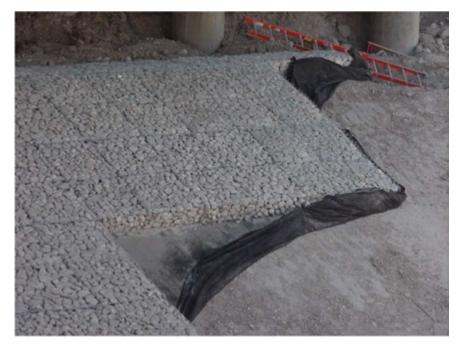
Figure 13-15: Gabion Mattresses at Bridge Abutment
