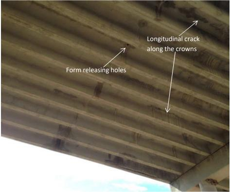
Figure 4-5: Longitudinal Cracks on pan girders.
