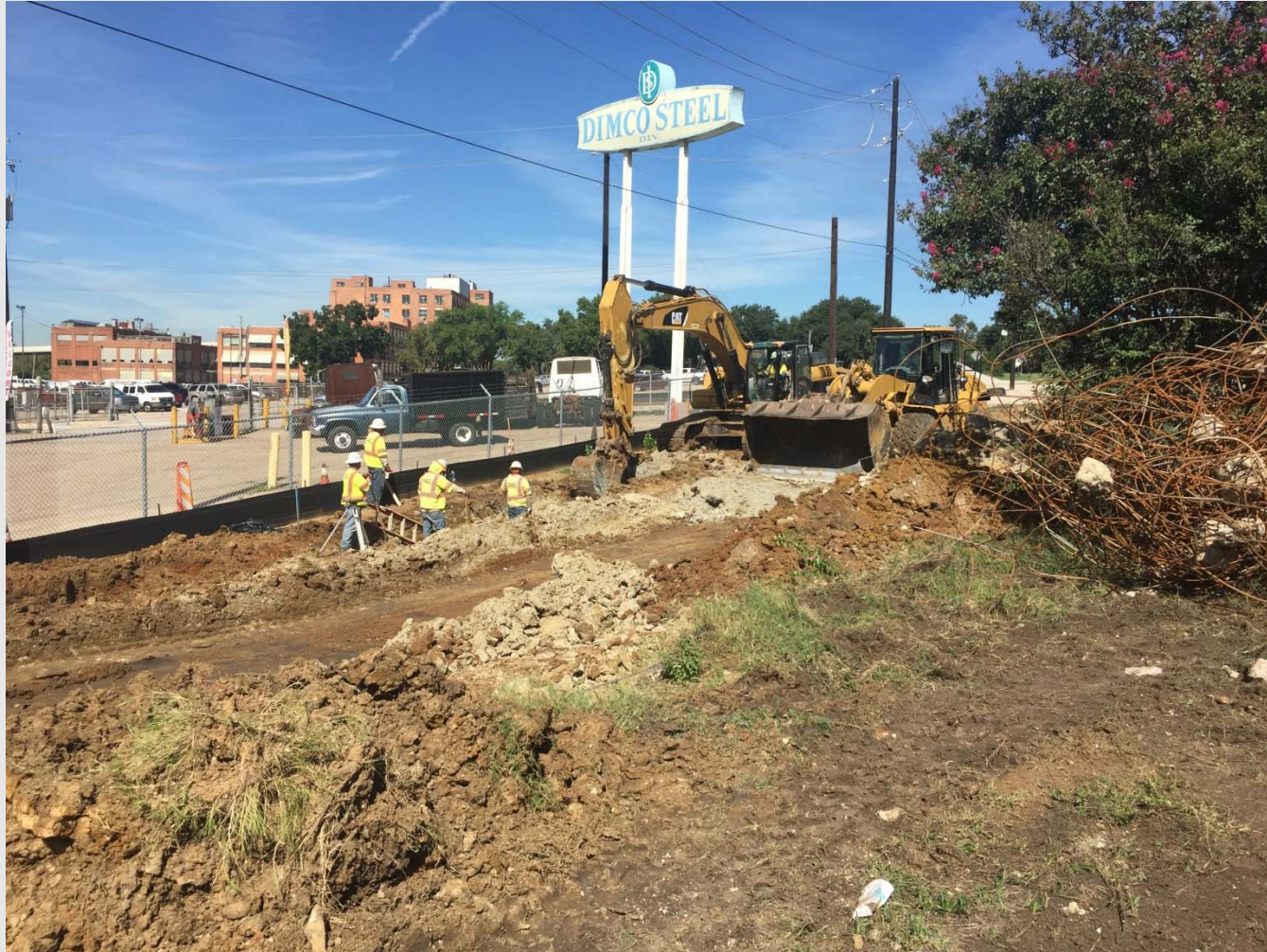
Water Line Installation Work
