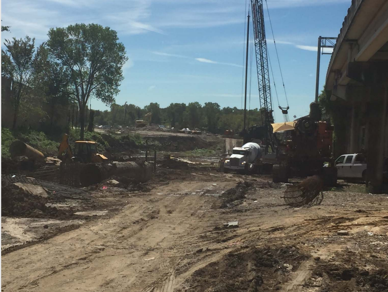
Drill Shaft Foundation Work – Northbound US 175 to Northbound IH 45
