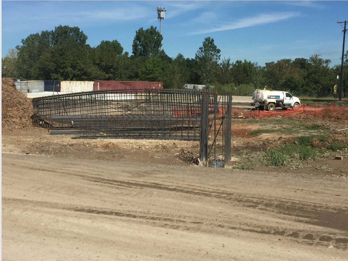
Bridge Foundations - Southbound IH 45 to Southbound US 175 Bridge
