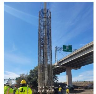
ANC Drill shaft construction at I-35/I-410 N interchange
