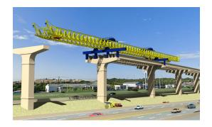
than half of the girders with launchers. When using this state-of-the-art method, no major cranes will be needed. ANC will self-perform the launching scope with specialized crews. We have partnered with the equipment manufacture to design and provide the heavy-lift equipment. This addresses the resource limitations of a very competitive and busy market.
