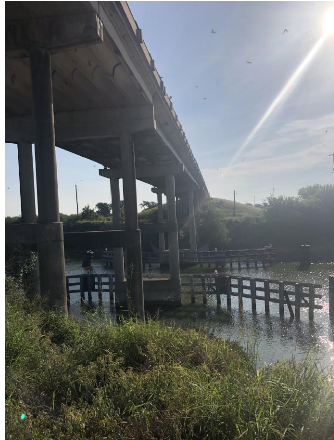
Figure 2-1 | Bridge and Fender System
