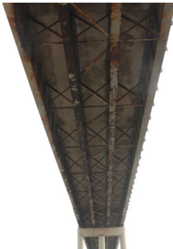
Figure 4-1 | Underside of the Superstructure
