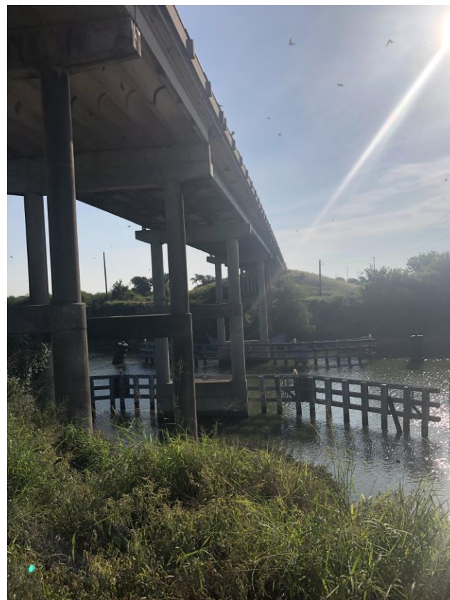
Figure 2-1 | Bridge and Fender System
