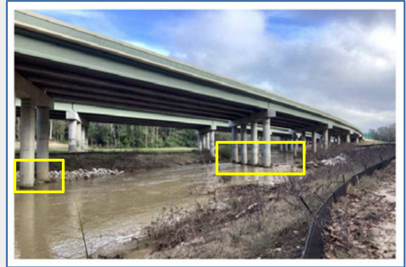
Latest Inspection Photo: New bridge with no Scour
