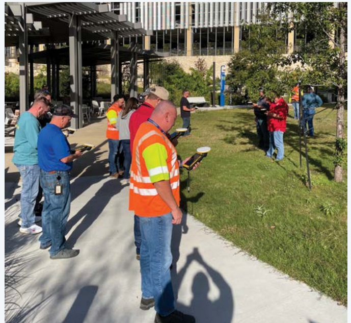
Employees test out their new surveying equipment at a training session in Austin. Photo provided by the Engineering Services Delivery team
