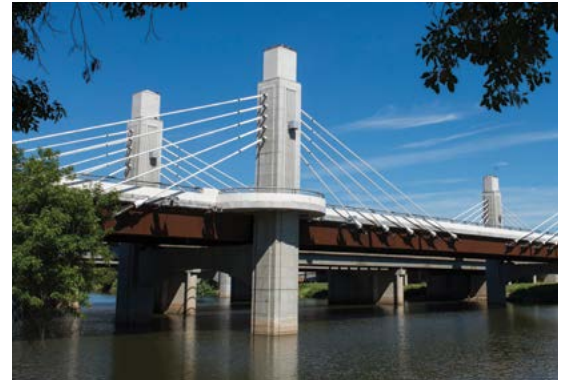
TxDOT was named Owner of the Year for its implementation of steel bridges like the Brazos River Bridge in Waco. Photo by Michael Amador
