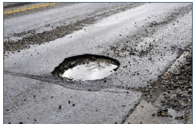
Figure 2: Existing Project Pavement and Bridge State of Repair
