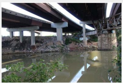
NOTE: 1. North channel bank is steep and has moderate scour due to channel bank and run-off erosion. Rock rubble riprap has been previously placed to provide protection and control scour but due to steep north channel bank some rock rubble has partially settled in the channel bed.
