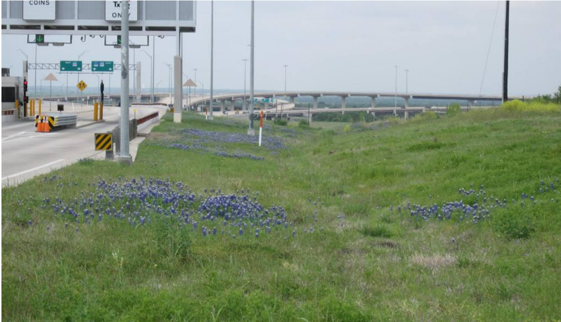
Figure 7 – Desired Shoulder and Turf Condition
