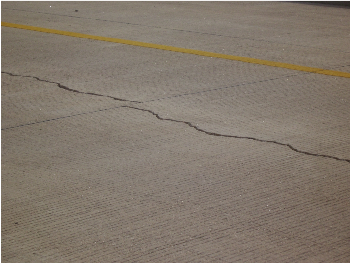
Figure 4 – Pavement Crack on Loop 1
