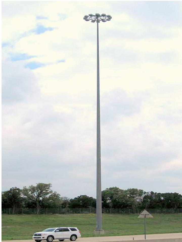
Figure 15 – High Mast Light Tower
