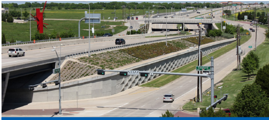
NTTA's DNT 463 project in Frisco, TX was led by our PM, Ben Withered to a successful on-time, under budget completion
