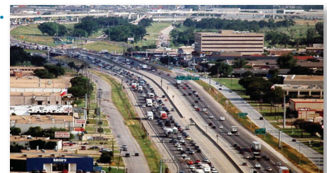
IH 35E Managed Lanes Design Build (IH 635 to US 380)
